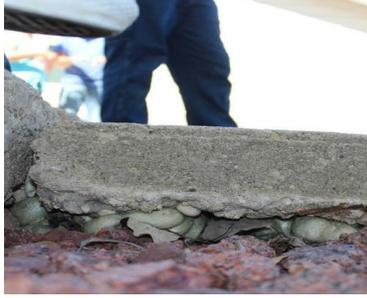
**Poor or improper compaction of the base before concrete was poured:** The weight of the slab will further compact the base after curing, and settlement can happen quickly.
