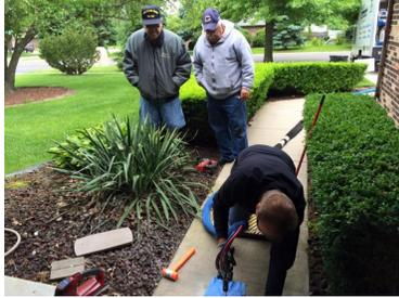
mudjacking with dirt, water and cement mixture to raise concrete slabs: driveway, sidewalk, patio, and porch or pool deck. Joe is the expert in doing the work. Pictured here is Joe, working on a sidewalk repair! Small jobs are not a problem for us! Our concrete raising solution is a cost effective, eco-friendly, time-saving alternative to traditional mudjacking. With our Polyurethane Foam, you won't have to raise your concrete again!
