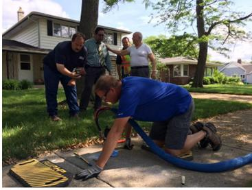
Polyurethane Concrete Raising and Mudjacking are both techniques used to repair settled concrete by lifting the surface back to its prior position. The core processes are very similar, but there are several advantages of using Polyurethane Foam over Mudjacking despite the higher cost. To understand what makes it better, one needs to know the difference between both the techniques.
